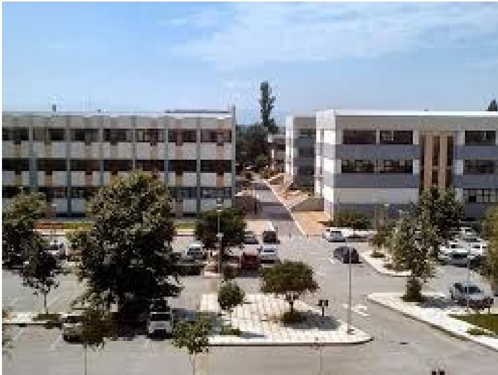
Figure 1. View of the Department's building, where Auditoriums, Classrooms and Laboratories are located
